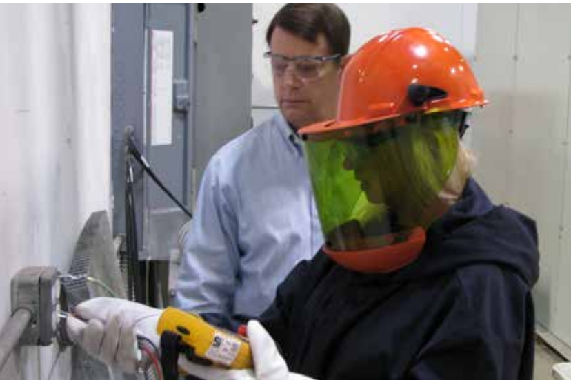
Verifying Meter Operation for a 208 V MCC
